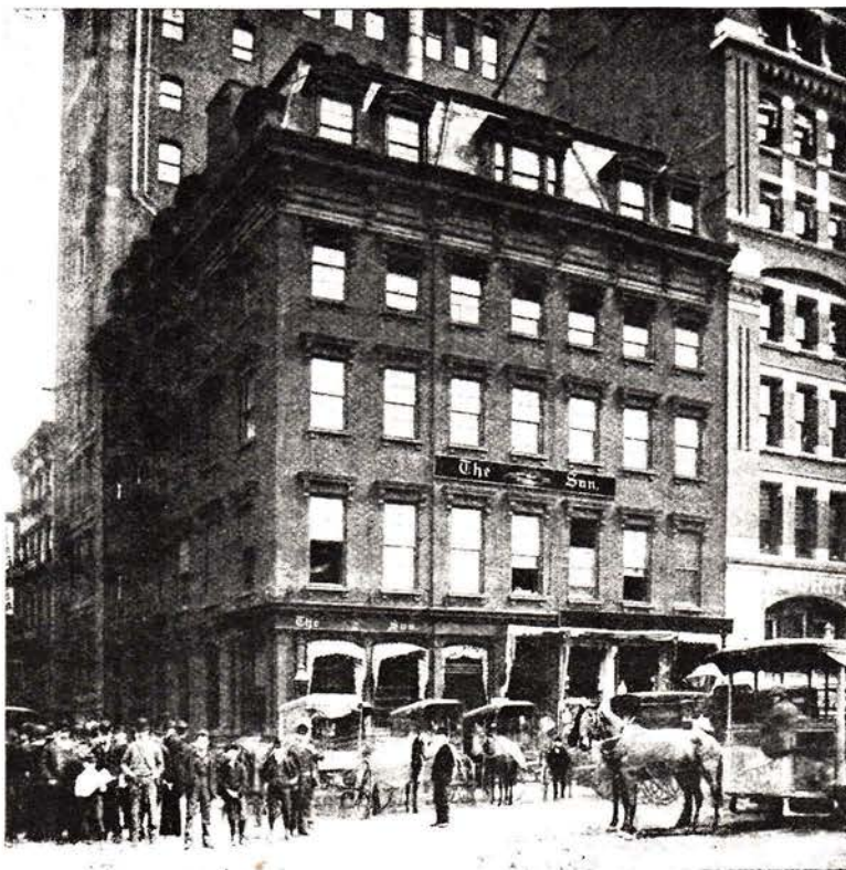
THE BUILDING ON NASSAU AND FRANKFORT STREETS.
