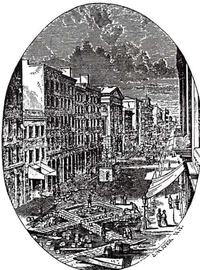
Laying the Russ Pavement in Broadway, corner of Reade-street.
