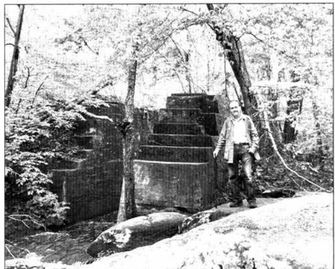
H.A.S. convention host Jack Bales stands next to an abutment designed to carry railroad tracks over a stream. Plans for the Fredericksburg, Virginia, railroad were made in the 1850s, but the Civil War interrupted progress and train service did not begin until the 1870s. The concrete abutment shown here dates back to the 1920s.
